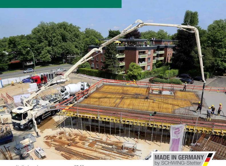
Vertical reach 37.30 m Concrete output 162 m<sup>3</sup>/h max. 85 bar Pressure on concrete max.
