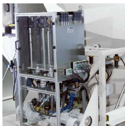
Admixture weighing system for chemical additives.
