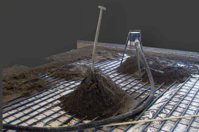
Sand, cement, water and additives are fully automatically mixed and transported to the workplace.
