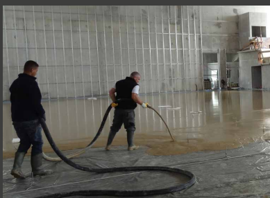
Precise material dosage allows the production of homogeneous and high-quality self levelling floor screeds.
