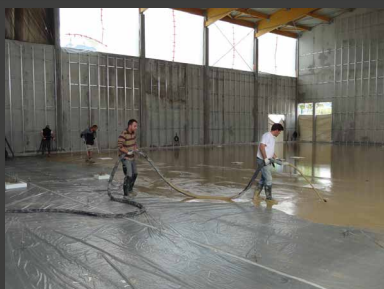
The precise material dosage guarantees the production of a homogenous and high-quality self levelling floor screed.
