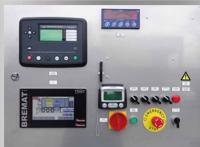
The computer controlled system is equipped with an advanced touchscreen display and is easy to operate.
