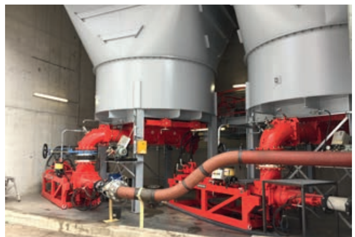
Pumping of dewatered sewage sludge in a cement plant Germany
