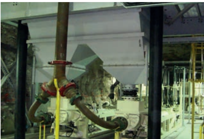
Pumping of mining residues in a diamond mine Canada
