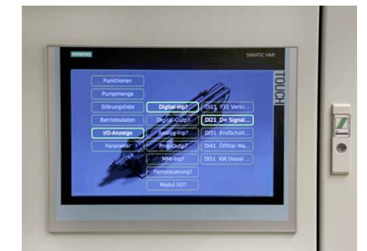
Touch panel on PLC control unit for operating the sludge pumping system
