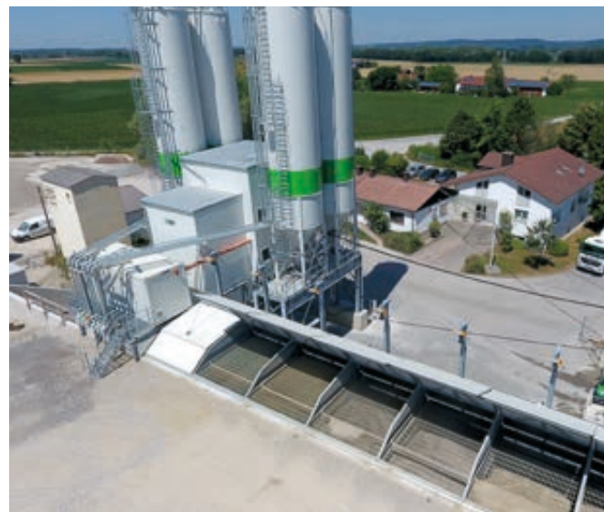
Quality assurance: gratings to protect against oversize grain
