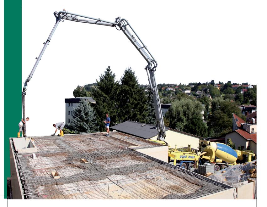
With its lightweight construction, SCHWING is able to achieve a total weight of less than 18 t, without making any compromises in respect to the core pump battery, Rock valve and boom.
