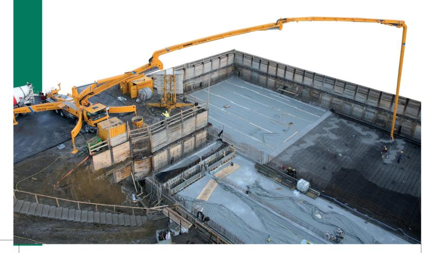
Only SX outriggers free up enough space in the machine's substructure to accommodate a pump kit with a stroke length of 2.5 m. These long-stroke pump kits, proven in many years of operation, are an ideal match of diameter and stroke.
