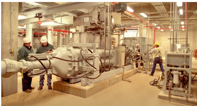
WWTP Blue Plains, Washington, D. C., USA
