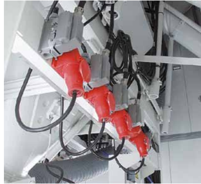
Plug-in connectors for the electrical connection of the peripheral devices make assembly and disassembly operations easier.
